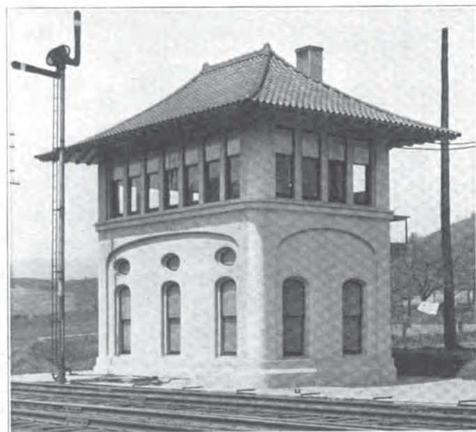
Fig. 2. View of Tower.
