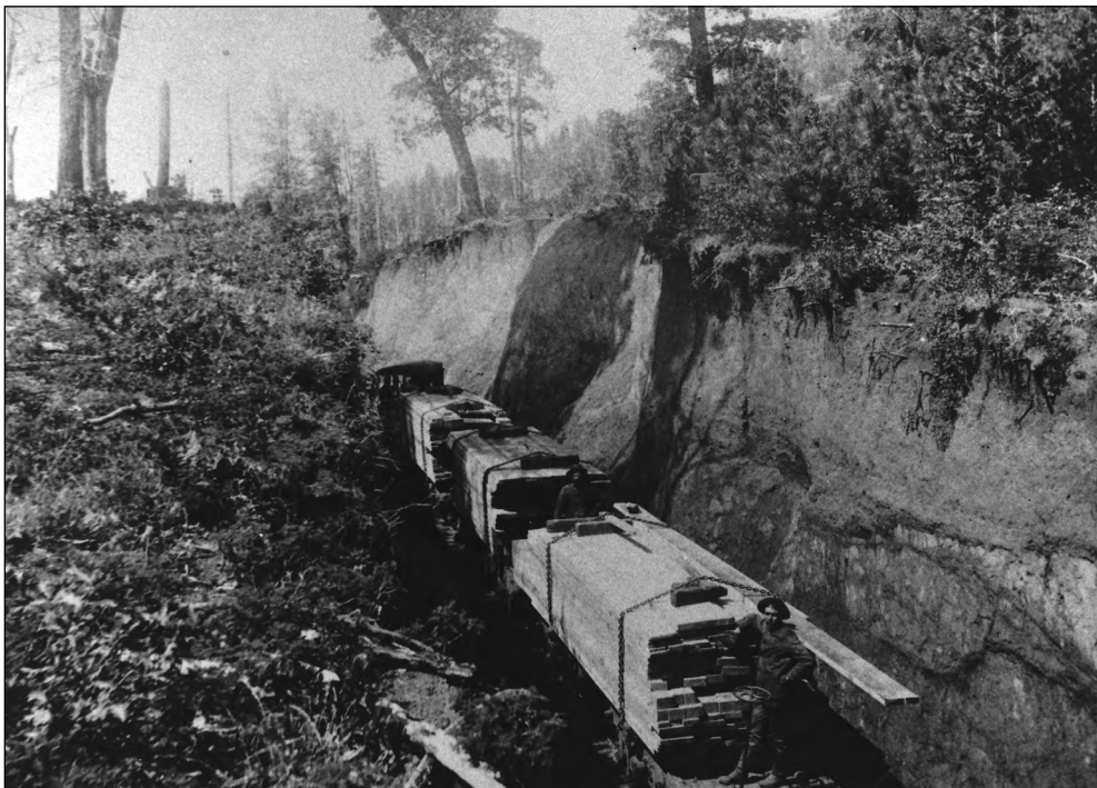
Figure 12—Numerous cuts and fills were needed to maintain the rail grade from the Beanville mill to the Challenge flume.
