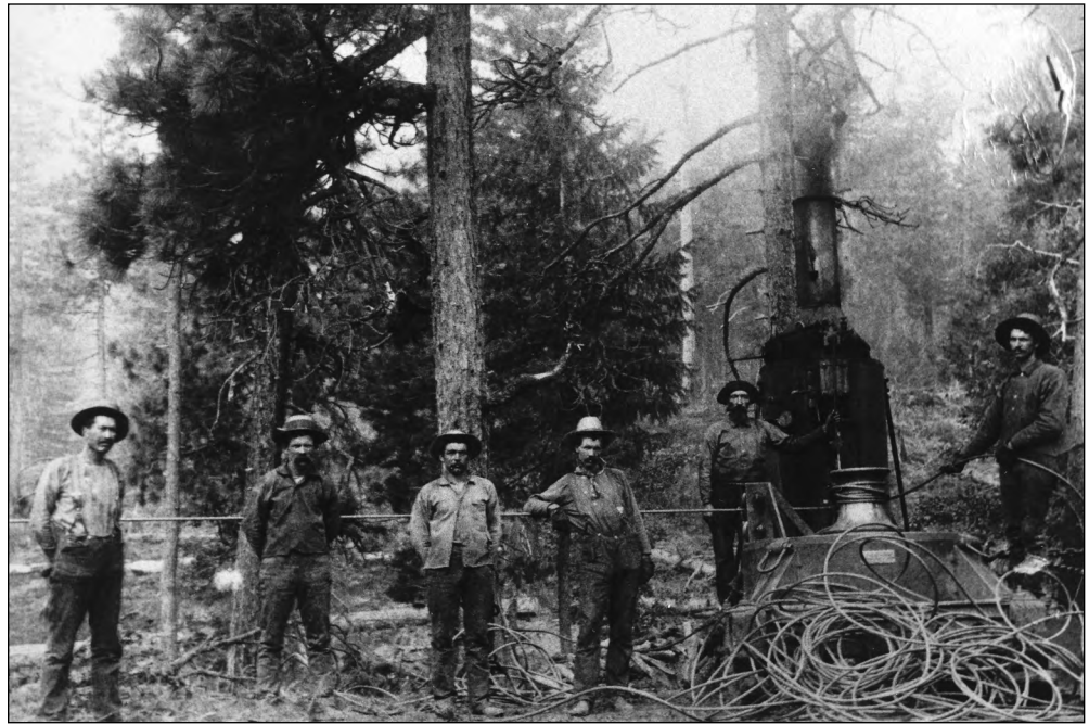
Figure 13—This little, wood-burning, steam donkey engine and crew snaked logs out of the woods enroute to the Beanville Mill in the early 1890s.
