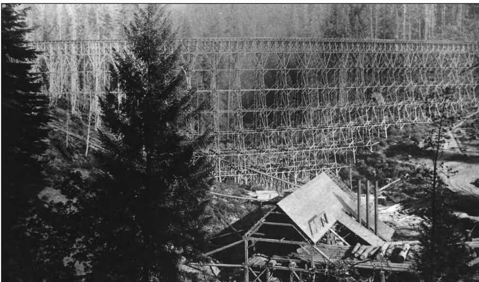
Figure 9—To flume across Owl Gulch creek and canyon, a trestle 166 feet tall was required. Note the mill and typical size of logs in the foreground. Although unknown, a tramway probably carried the lumber to the flume.
