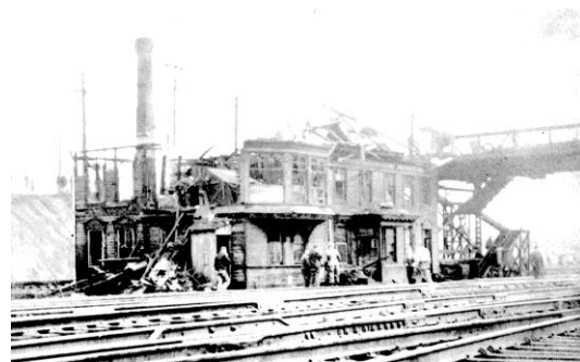
ROSE TOWER-Juniata- March 28,1953 following damage by fire. Seven employes on duty at the time escaped uninjured.
