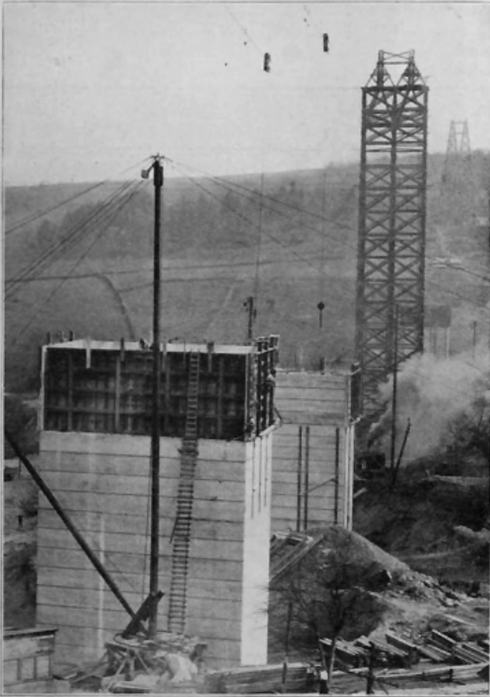
Showing Sectional Pier Forms and Double Cableway.
