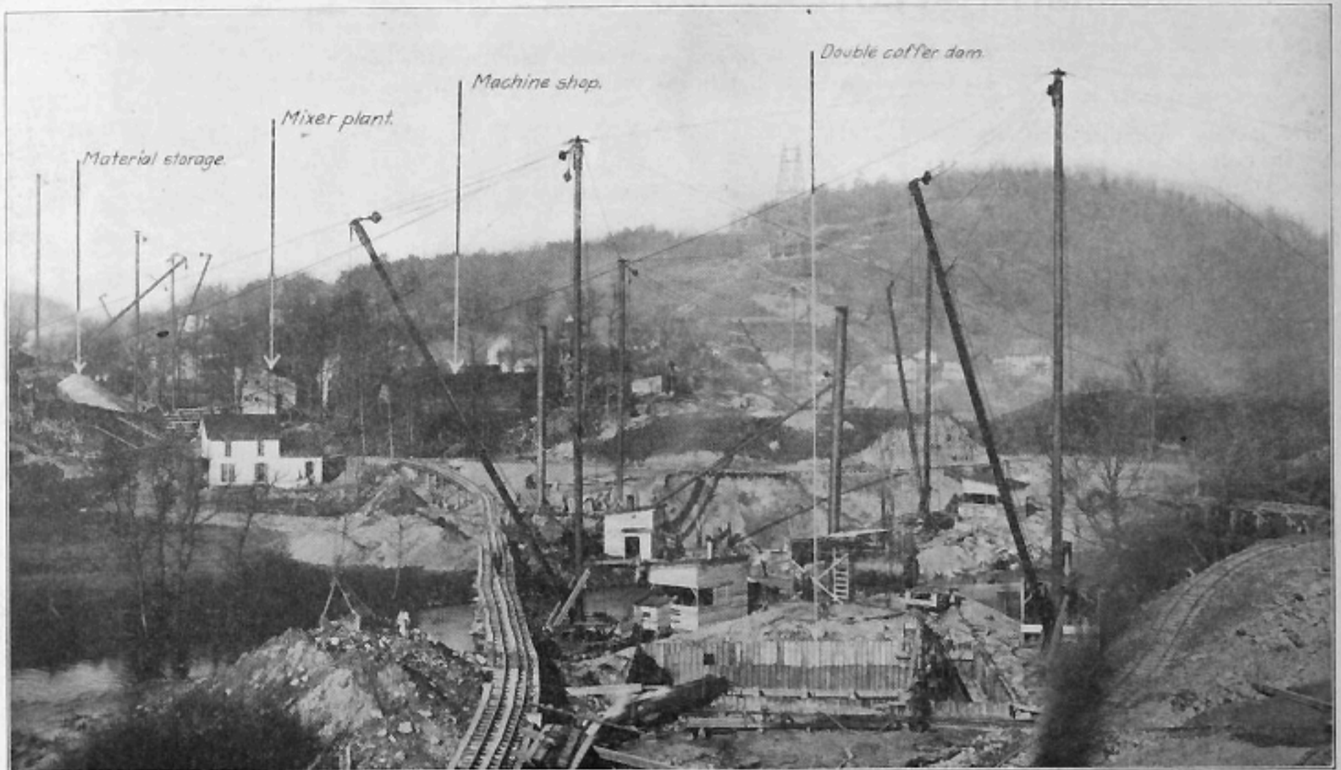
Looking Along Center Line of Tunkhannock Viaduct in Early Stages of Construction.
