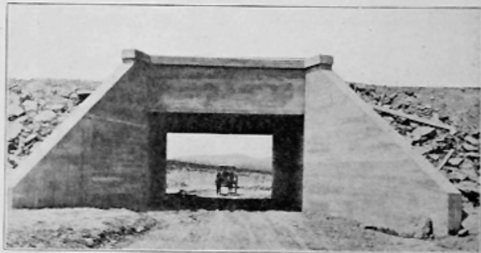
A Typical Highway Undercrossing.
