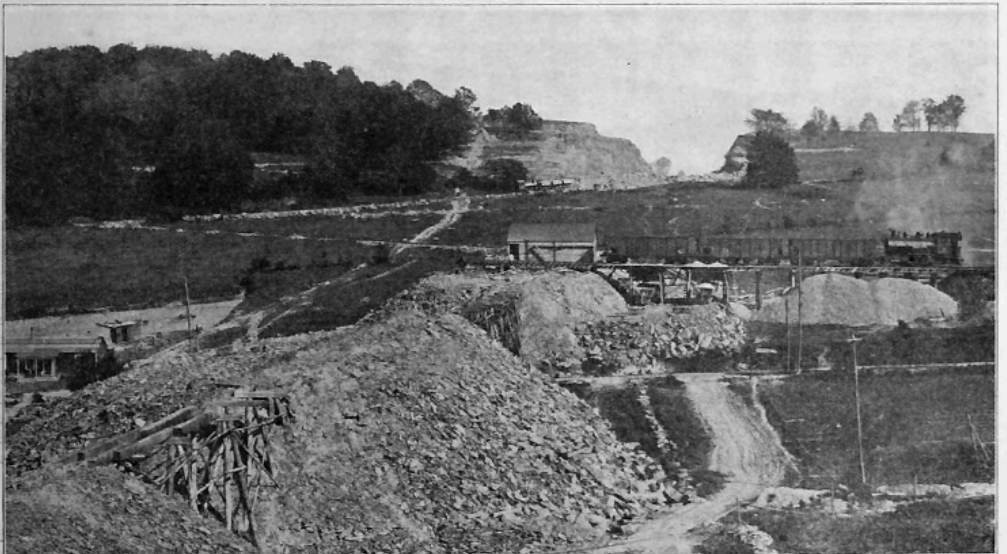
Slayton Cut and Switchback to Fill in Foreground.
