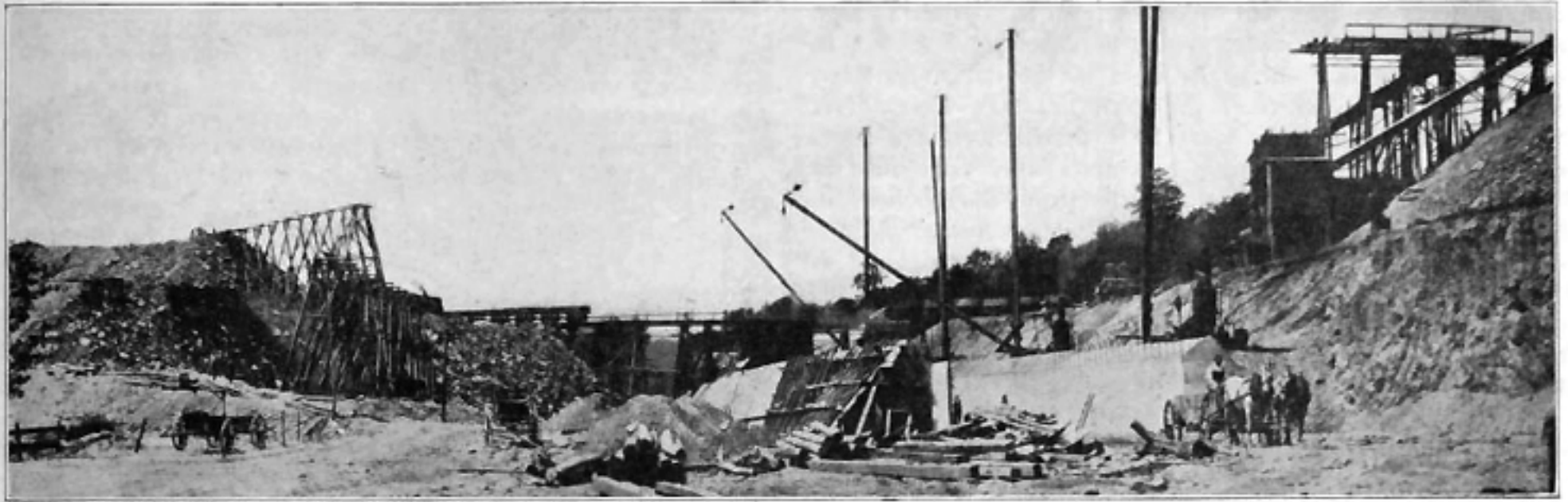
Smith Fill Under Construction Showing Two Heights of Trestles.
