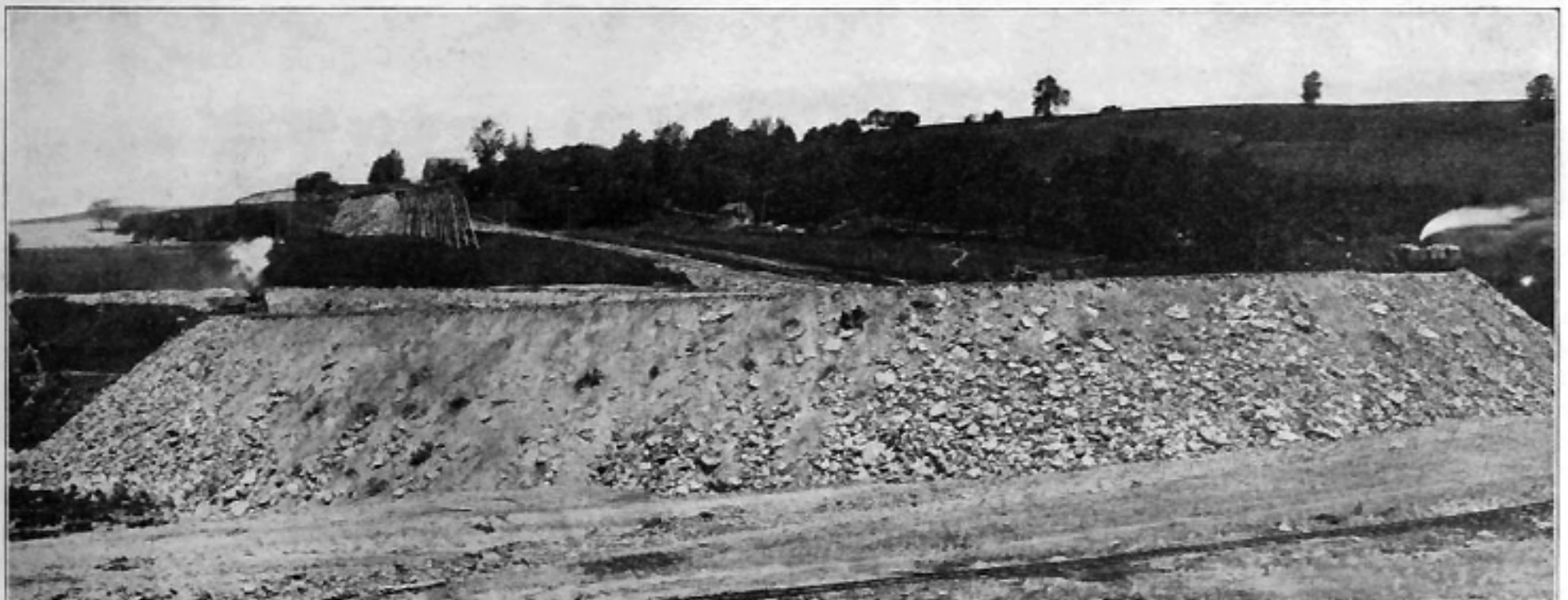
South Branch Fill, Showing Balanced Incline to Lower Lift and Upper Level Trestle.
