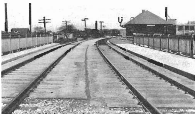
View Showing Deck and Track Construction on the St. Clair Avenue Bridge
